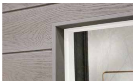
Fig 14 - Window/door head with mitred joint
